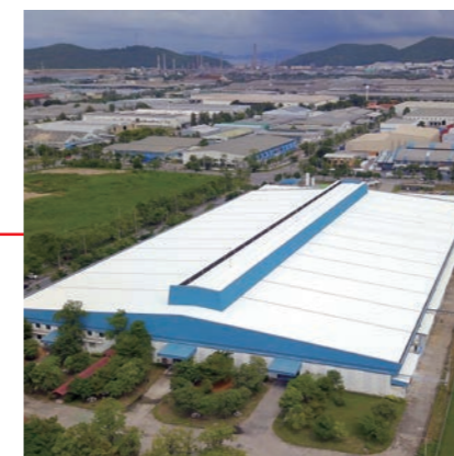
Fujitsu General (Thailand) Co., Ltd. (Thailand) Factory-2
