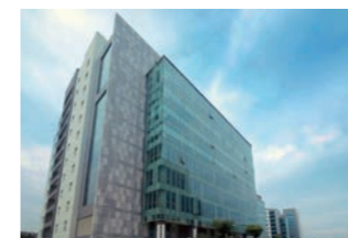
ABS Aircon Engineers Private Ltd. (India)
