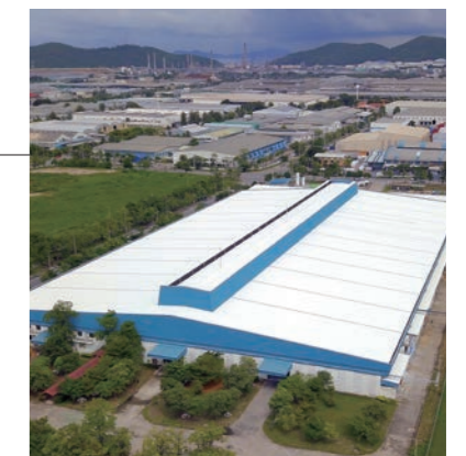
Fujitsu General (Thailand) Co., Ltd. (Thailand) Factory-2
